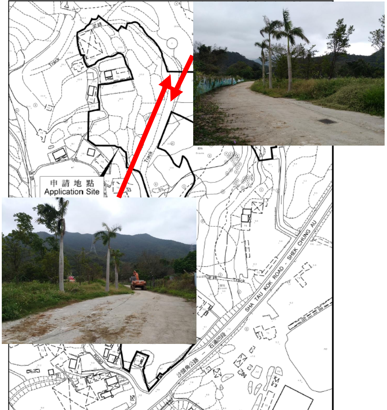
Figure 2 The proposed road has already been built in the site before submission of this planning application
