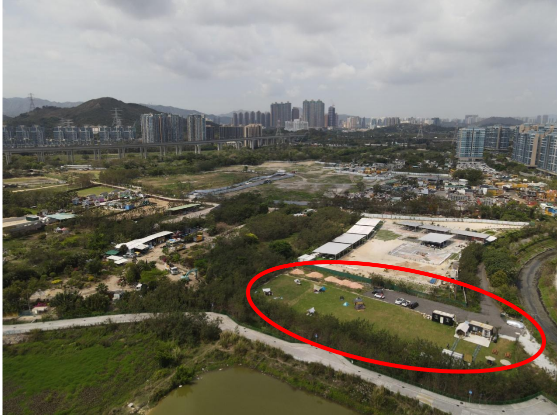
Figure 5 Site condition observed in mid-March 2021 (circled in red)
